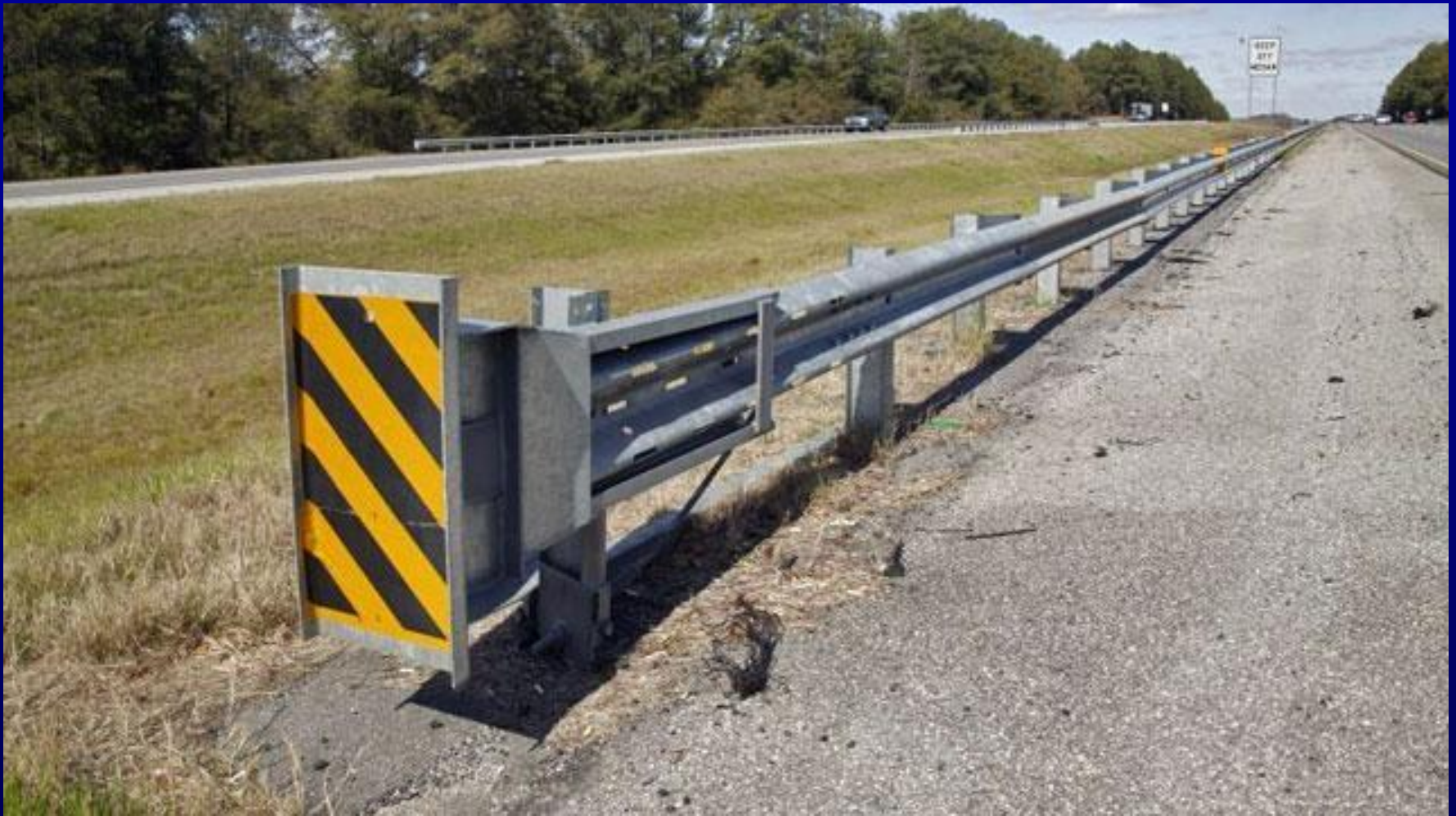
Energy absorbing guardrail end treatment
