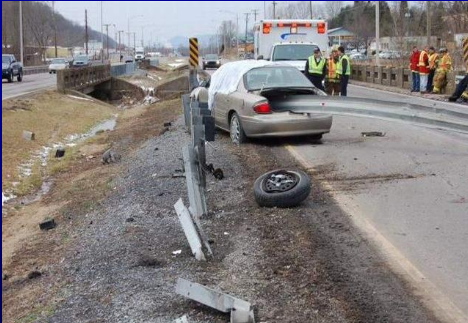
Blunt guardrail end treatment
