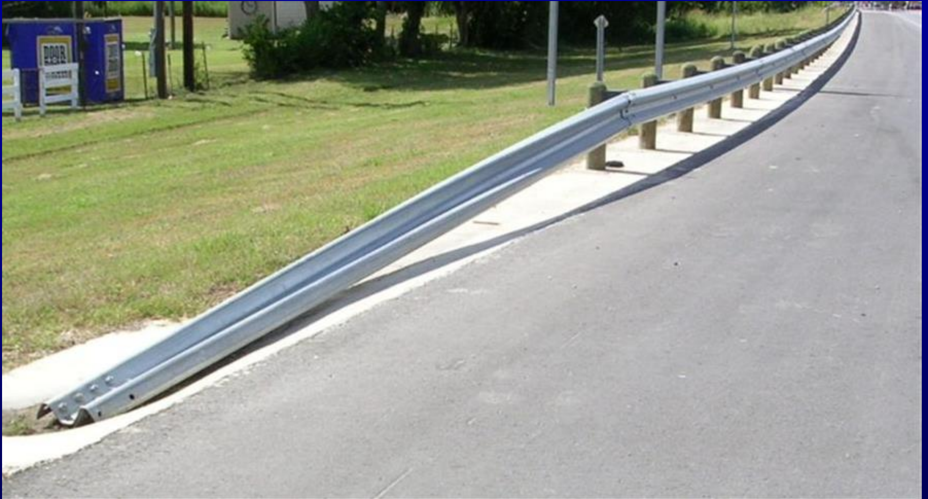
“Turned Down” guardrail end treatment
